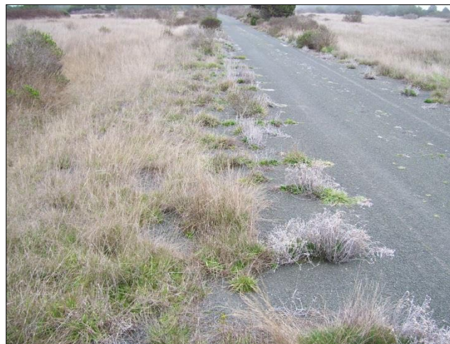
Figure 1.4 Example of Rural County Road
